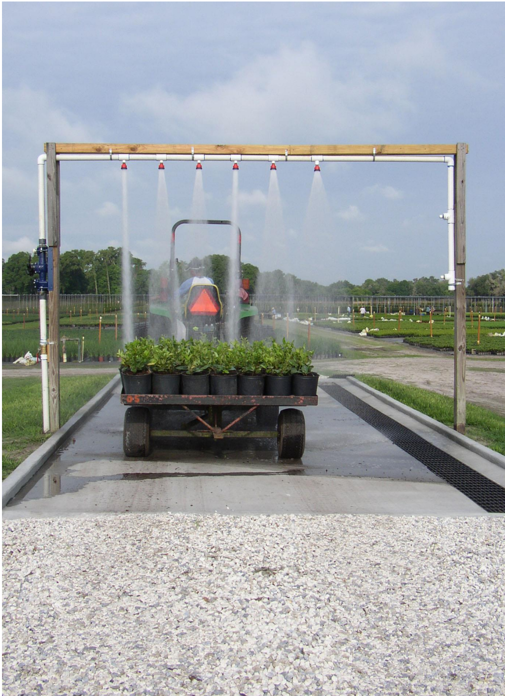
Figure 4. Photo of concrete pad installed for runoff management.
