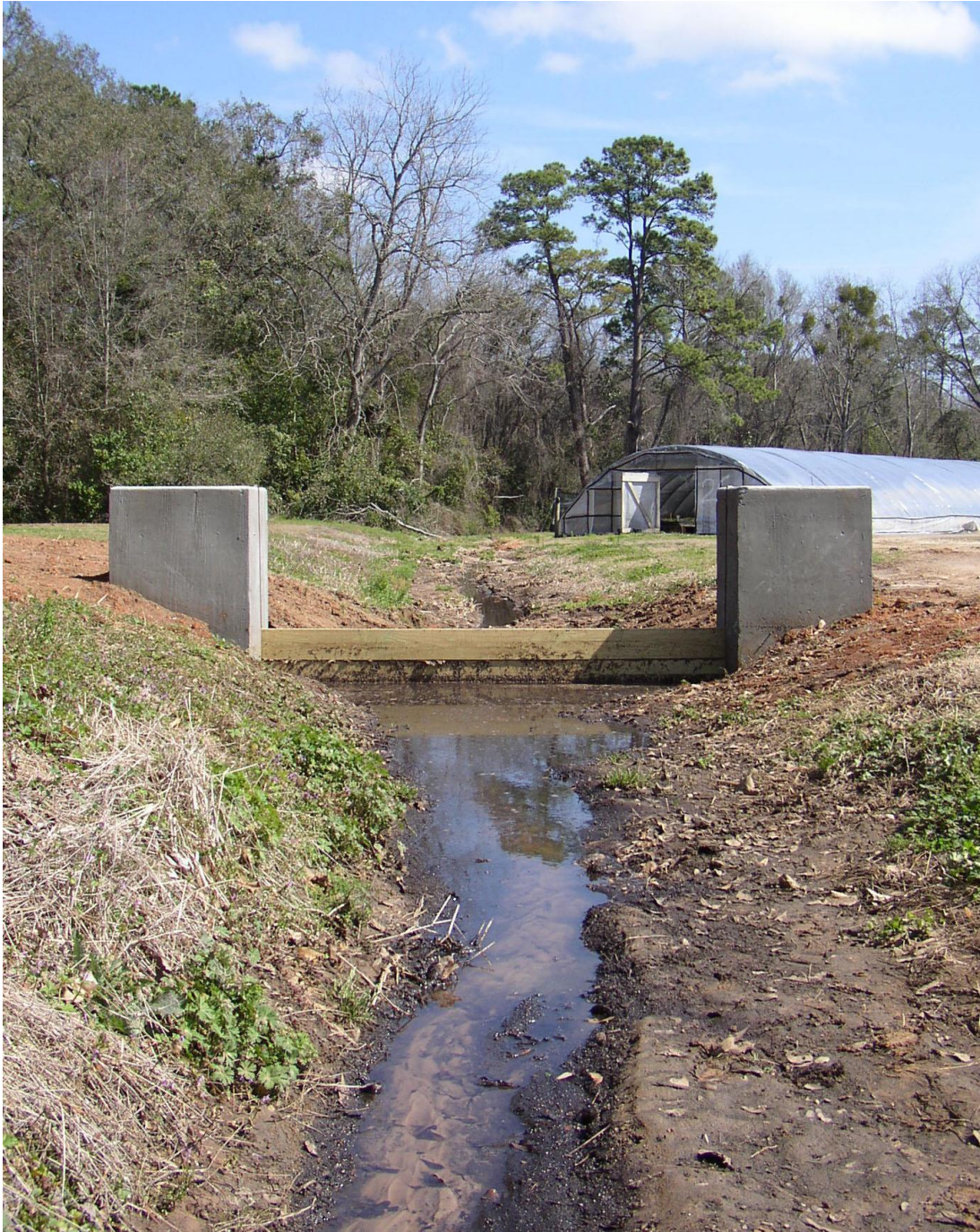
Figure 2. Photo of wall installed for runoff management.
