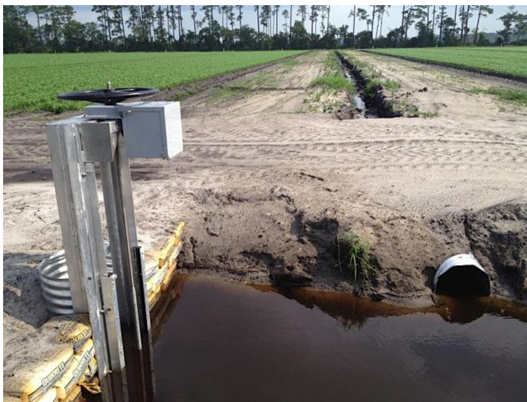
Figure 8. Water retention structure installed in tail water ditch and drainage ditch feeding into tail water ditch. Summer cover crop planted in the new research area.
