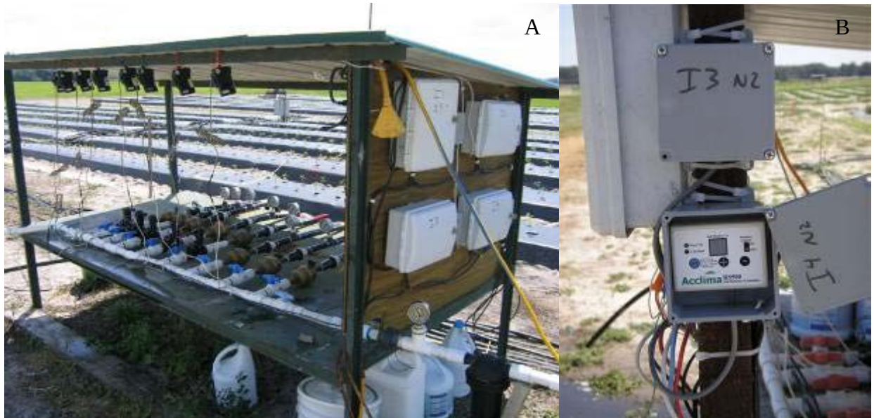
Figure 5. A) Experimental irrigation monitoring manifold showing flow meters, solenoid valves, and pressure regulation B) Acclima RS500 soil moisture controller.
